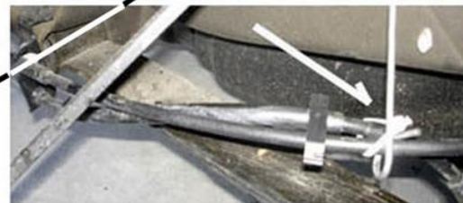
ensure cables are clear of installation
